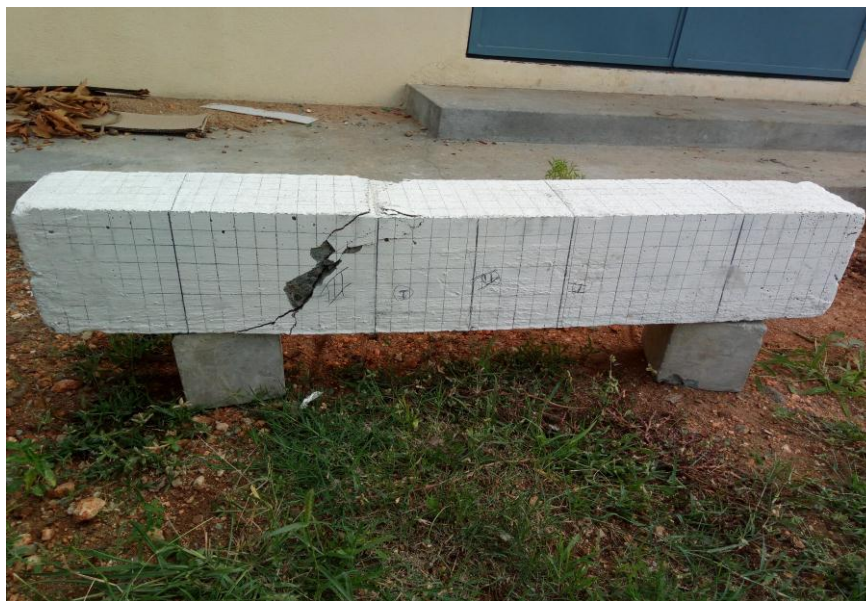
Fig. 4 Beam specimen after testing
