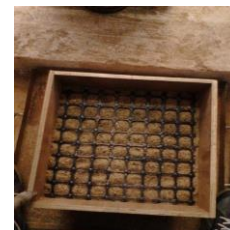
Picture 4.2: Placing of Geogrid
