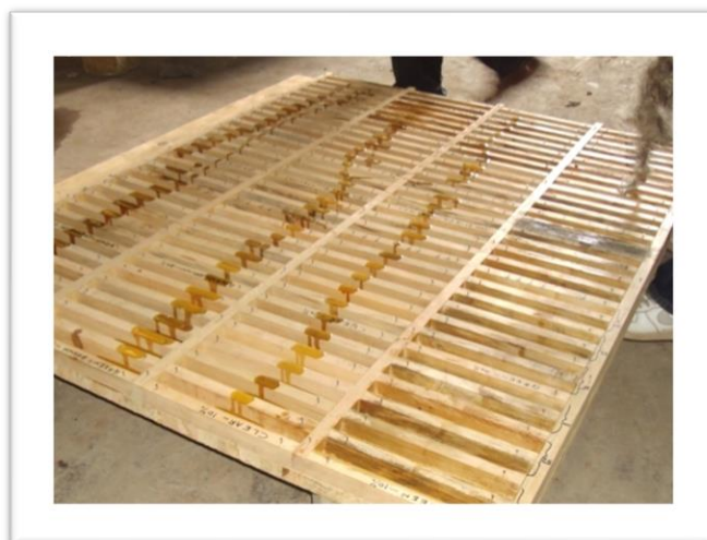
Plate 3.3b: application of the release agent
