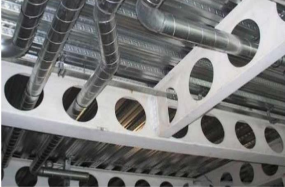
Fig.3. Service integration on beams through web openings [1]
