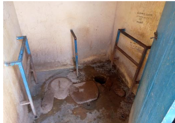
Figure 4: Steel grab bars (support rails) fixed to the floor and walls
