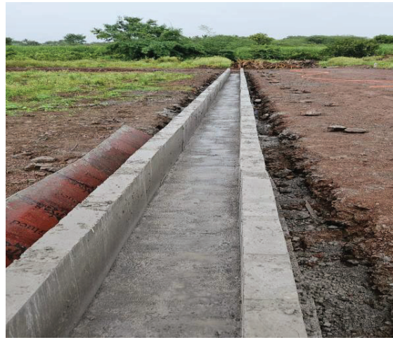
Figure 11 Drainage System Construction
