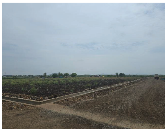
Figure 13 Construction of Water Bound Macadam Road
