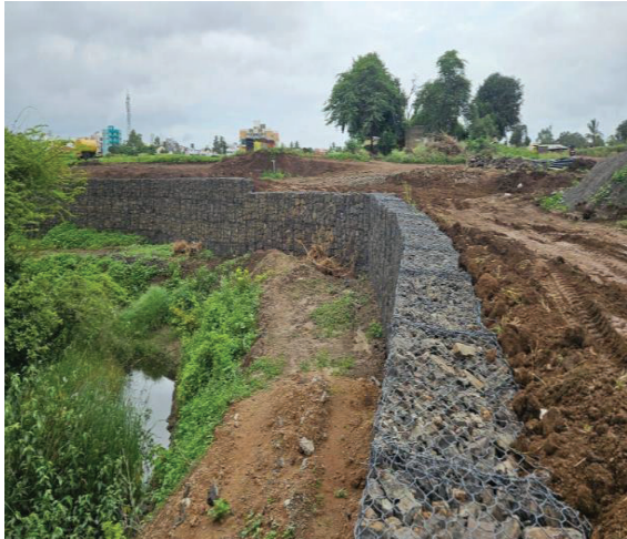
Figure 10 Gable wall construction
