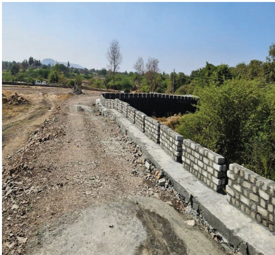
Figure 12 Compound Wall Construction
