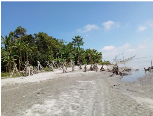
Fig 1: RCC Porcupines laid in Majuli, Assam
