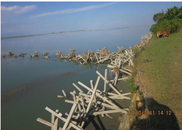
Fig 1: RCC Porcupines laid in Rohmoriam, Dibrugarh, Assam
