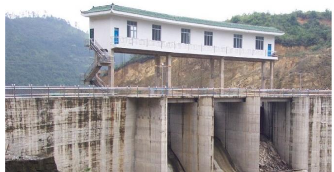
Fig. 1. Downstream view of Changsha Arch Dam [24]
