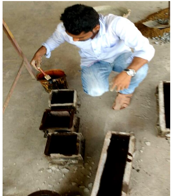
Fig 2 - Oiling of moulds
