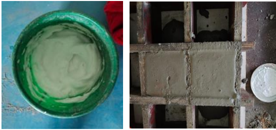
Fig 1: Casting of cube specimens
