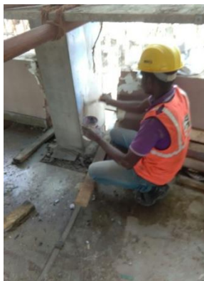
Fig 5 Applying AR compound
