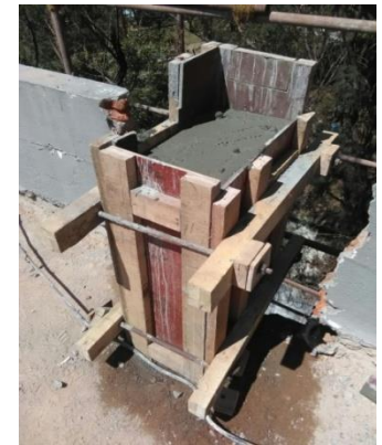
Fig. 4. Concreting with micro concrete
