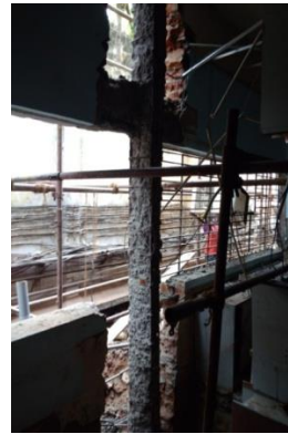
Fig. 1. Removing brick work
