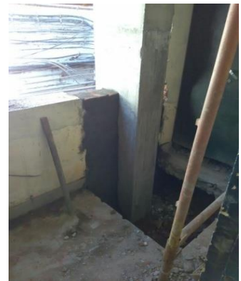
Fig 6 Redoing of brick work and plastering
