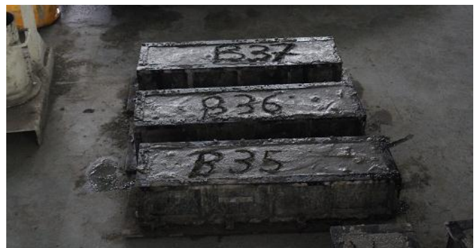
Figure 3: Casting of Beams
