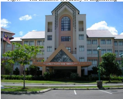
Fig. 2. The Façade of block A, Faculty of Engineering
