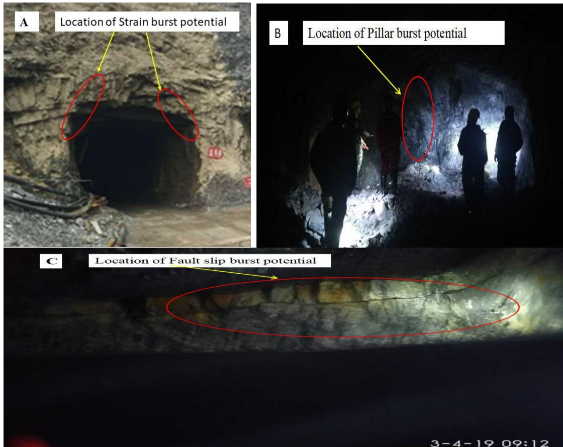
Fig 3. Presentation of the Location of rockburst potential (Strain, Pillar, and Fault slip burst mechanism)
