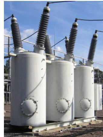
Fig. 7. Circuit breaker
