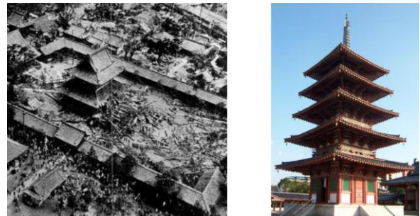
Figure 3: (a) Shiten'noji Pagoda collapse in 1937 and (b) Present day rebuilt structure
