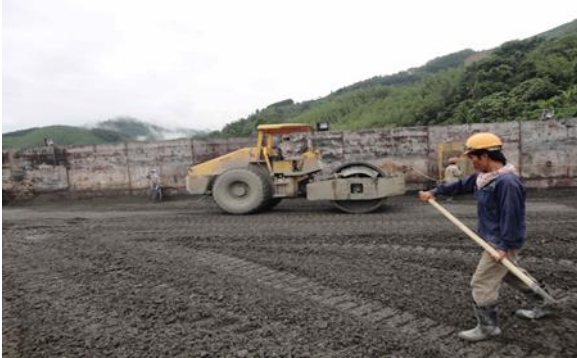
Figure 13. Compacting RCC by compactor, in hydropower project
