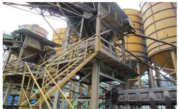
Figure 4. Roll-compacted concrete batching station
