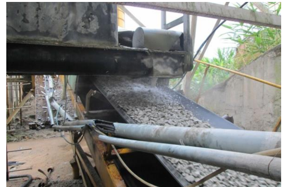
Figure 10. Adding ice to lower the inlet aggregate temperature
