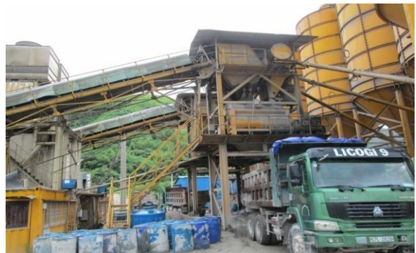
Figure 3. Roll-compacted concrete batching station
