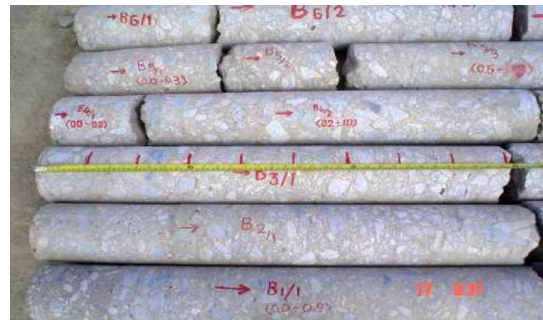
Figure 20. RCC drill core
