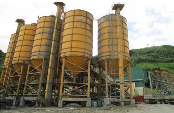
Figure 8. Cement and fly ash storage silos
