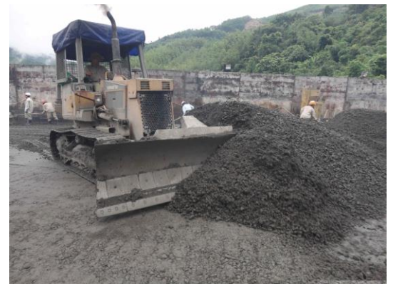
Figure 12. Leveling RCC by bulldozer in hydropower project
