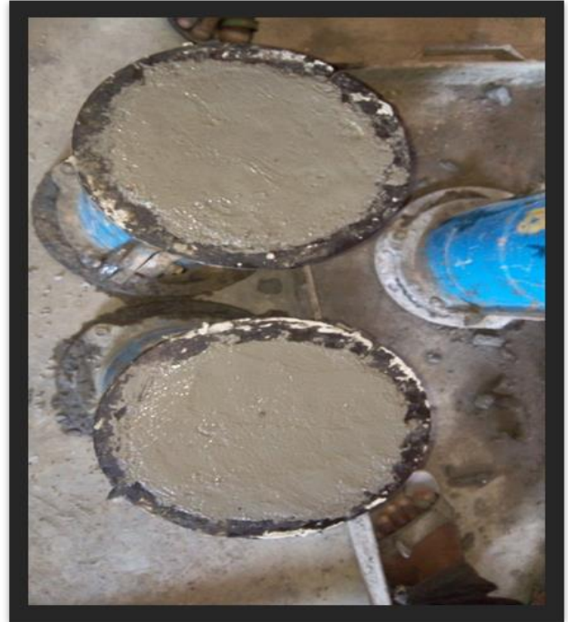
Fig. 4. Concrete Placing and compacting
