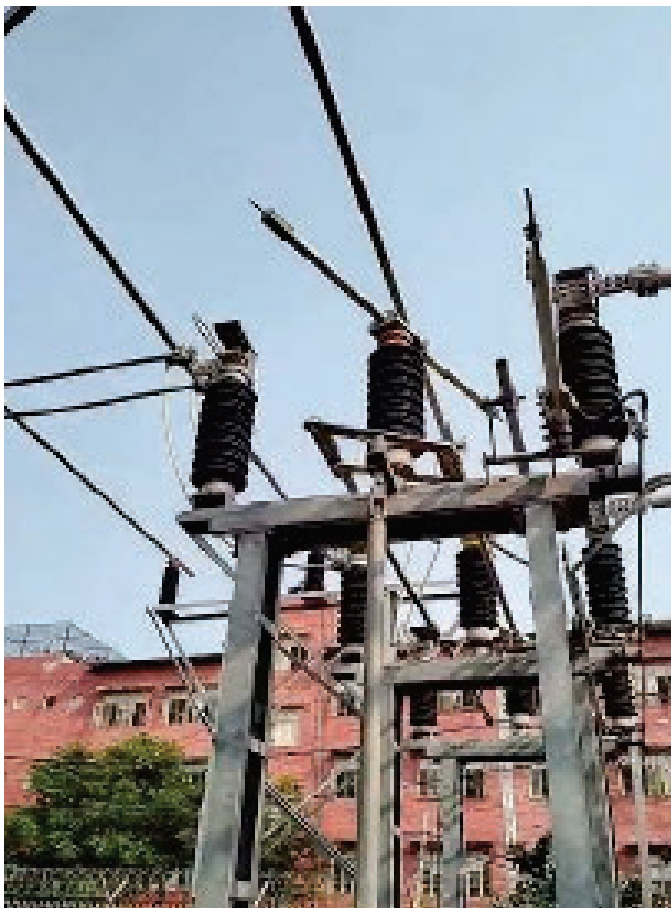
Fig. 2. Substation Isolator.
