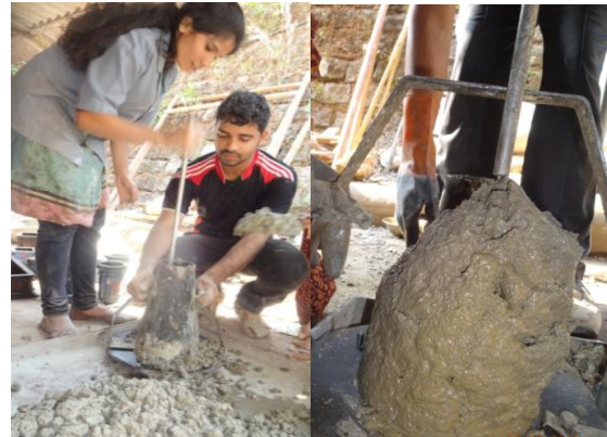
Fig 2: Slump test carried out on concrete
