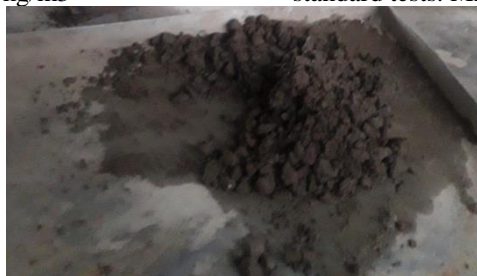
Figure 5 mixing of concrete
