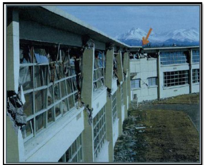
Fig. 1 - Damages caused to the roof diaphragm at the re- Entrant Corner of West Anchorage High School, Alaska, during 1964 Earthquake.
