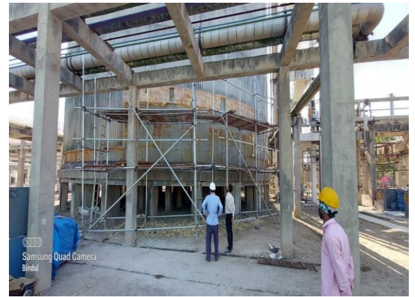
Fig 8. Removal of Shell insulation
