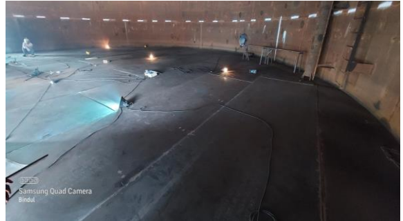
Fig 16. Final welding inside tank
