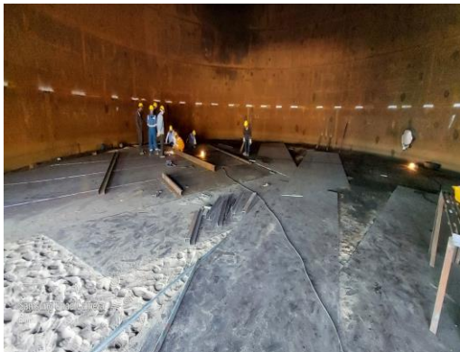
Fig 13. New plate welding started
