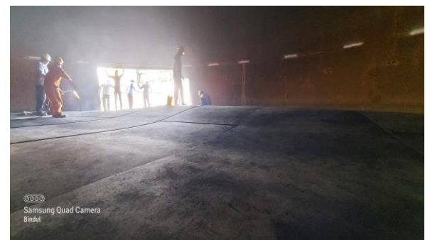
Fig 9. Removal of bottom plate
