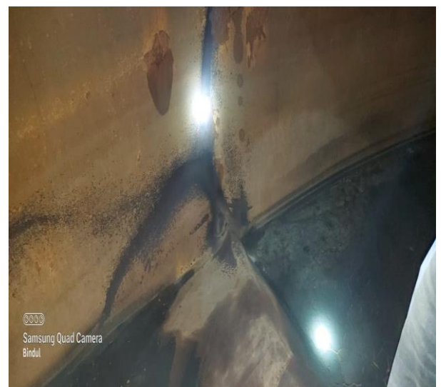
Fig 4. Bulging and through crack at bottom
