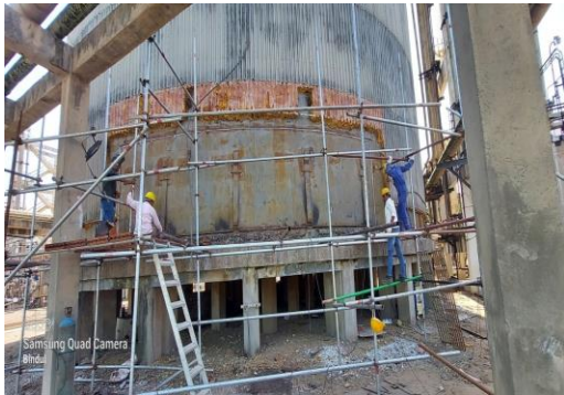
Fig 21. Final welding of outer tank shell
