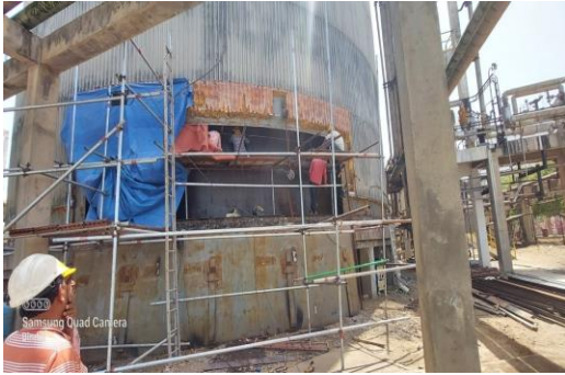
Fig 20. Final welding of inner tank shell
