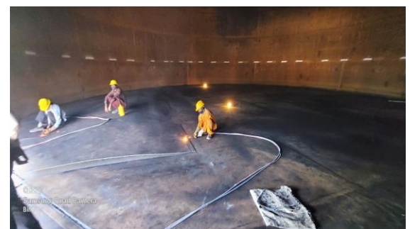
Fig 10. Cutting of bottom plate
