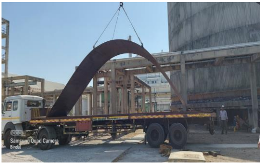
Fig 12. New plates unloading at site
