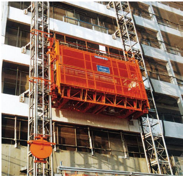
Fig 3: A low-voltage matrix converter is applied in an outdoor elevator for a building construction in 2011.
