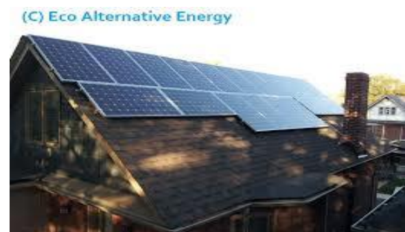
Fig.3: example for partial shading of solar panel
