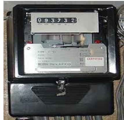
Fig. 1. Old analog electro mecanical electric meter
