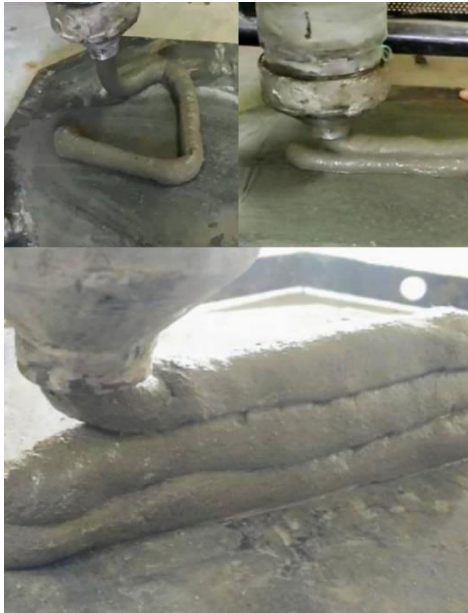
Fig 6: Layer formation using concrete extruder
