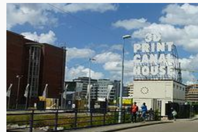
Fig 12. Printing 3D house project at Amsterdam
