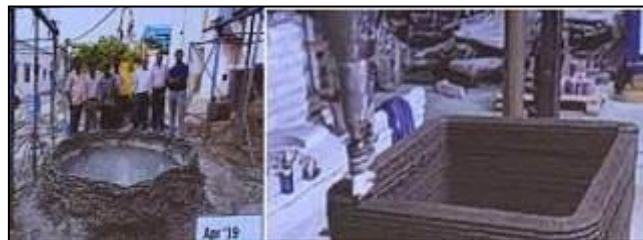
Fig -7: L & T has hand printed first water tank of capacity 2KL at Kanchi in year 2019 & First Trial with COBOD printer in year 2022
