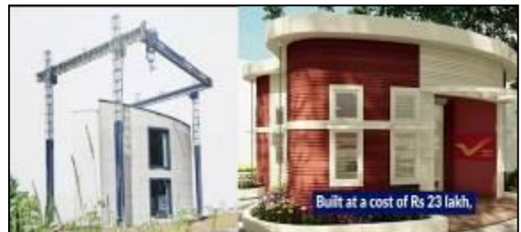
Fig -4: COBOD gantry type printer (BOD 2) & India’s first 3D printed post office building at Bangalore made with COBOD printer, constructed by L & T. 1000sqft in 45 days, Crew of only 5 peoples. Cost 23 lakhs. Life span 50 to 100 years
