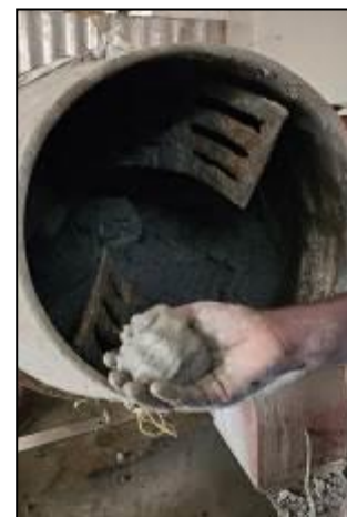
Fig -20: Trial Mix-01: Materials Mixed consistency checked
