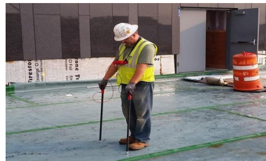
Fig.2. EFVM testing for leakage in roof
