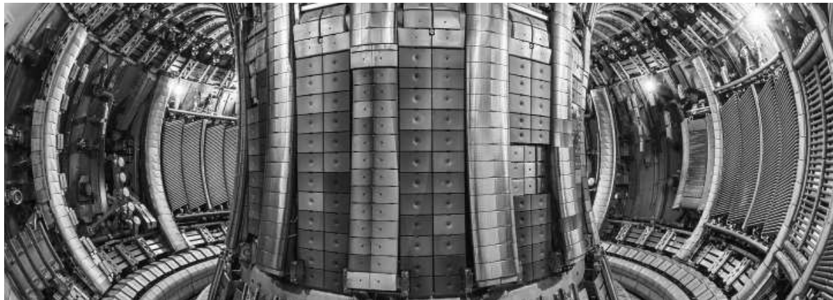
Figure 1.1: An internal view of the JET vessel with a complete metallic wall of beryllium and tungsten.
