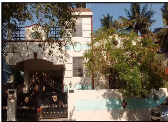
Fig 2 View of the existing building in Tambaram
