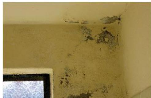
Fig.1. Image showing damages occurred in roof and wall due to water leakage
